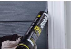
**19** From the interior apply OSI® QUAD® foam into the gap between the door and the framing. This must be a continuous seal with no visible shims.
